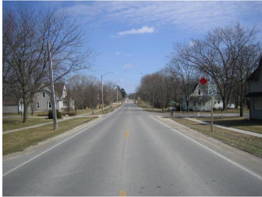
Figure 20: Site before converging chevrons
