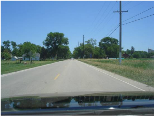
Figure 39: Site before surface treatment
