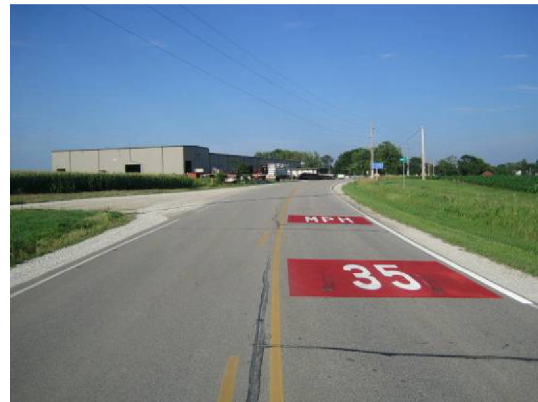
Figure 42: Curve after surface treatment
