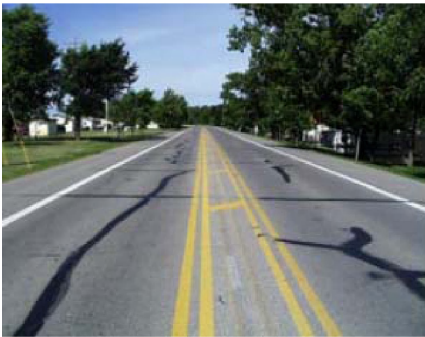
Figure 12: Lane striping to narrow lanes (30)
