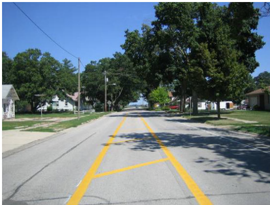
Figure 30: Site after lane narrowing
