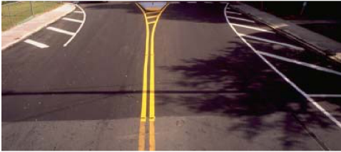
Figure 11: Lane striping to narrow lanes (41)
