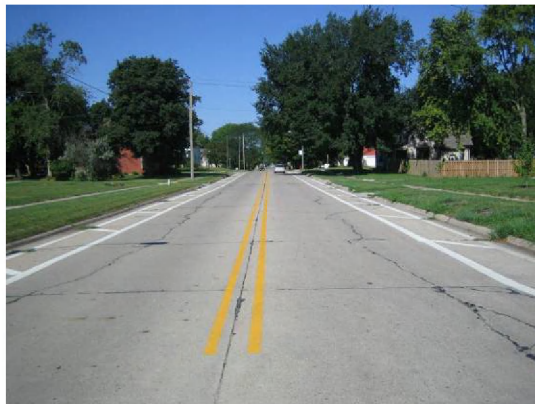
Figure 23: Site after lane narrowing
