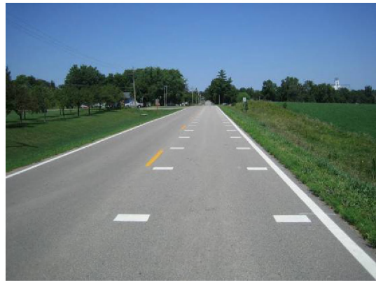
Figure 32: Site after transverse bars
