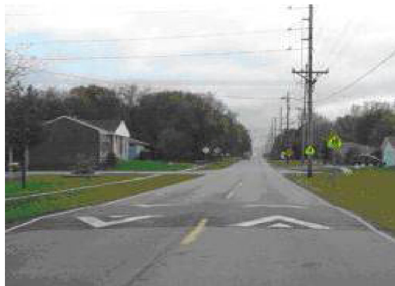
Figure 27: Site after speed table
