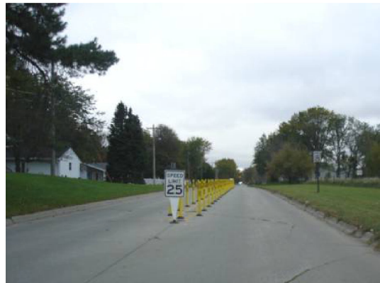
Figure 37: Site after longitudinal channelizers
