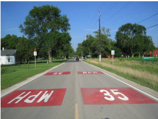
Figure 40: Site after surface treatment
