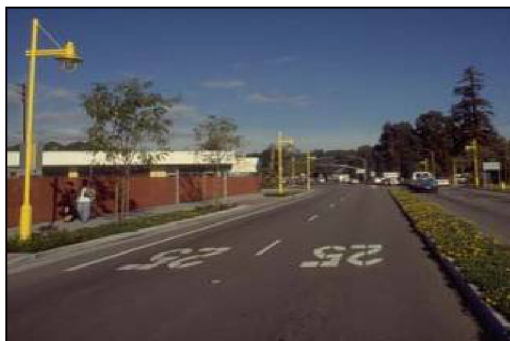
Figure 14: Speed limit pavement markings (41)
