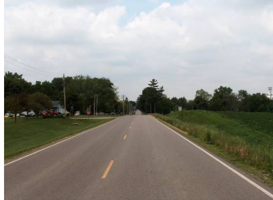
Figure 31: Site before transverse bars
