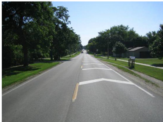
Figure 21: Site after converging chevrons
