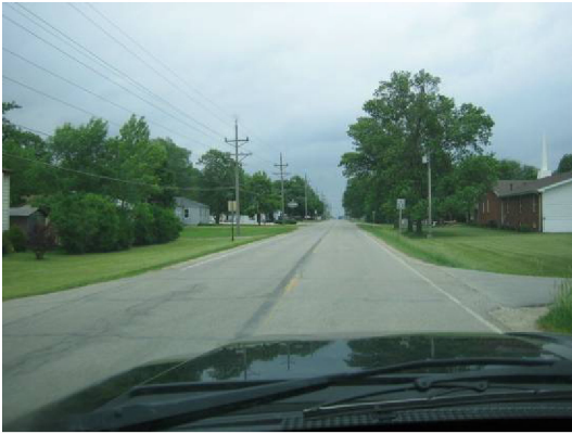
Figure 34: Site before surface treatment
