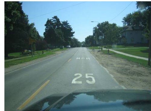
Figure 24: On-pavement speed signing
